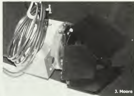
Above: Thousands of dollars were spent upgrading the lighting system in the studio. Workers had to install new electrical cables to the studio to handle the high amount of power needed for the lights.
